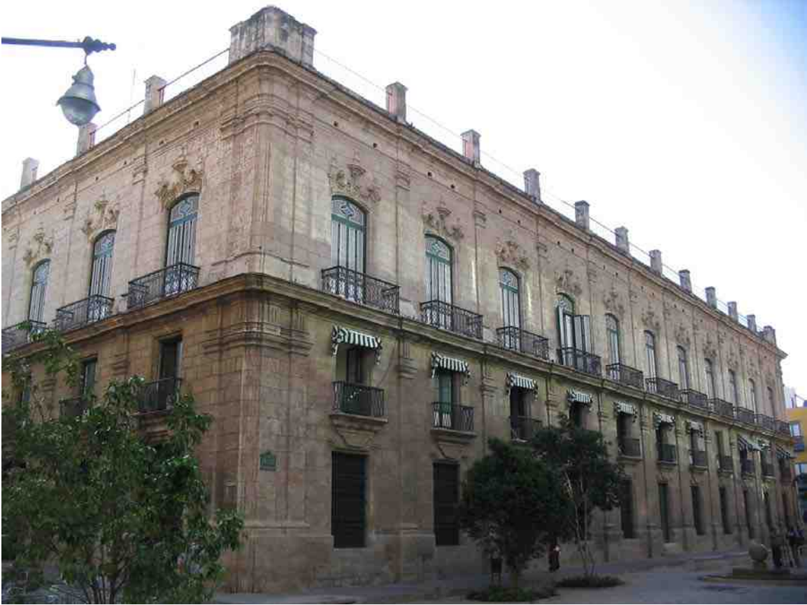
Figure 31. View of Palace of the Captain General from Mercaderes Street, Antonio Fernández de Trevejos and Pedro Medina, Palace of the Captain General, Havana, 1776-91
